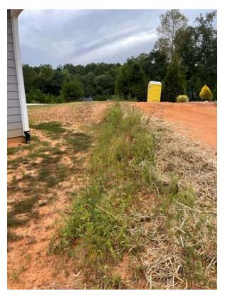
Sep '24 Resultant of our Drainage ditch/retention pool being filled with silt from Lot 7 runoff
