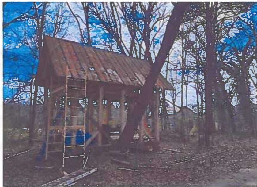
In January of 2025, we finished installing the roof of the restroom building.
