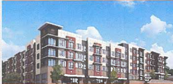
Clemson , SC (under construction)
