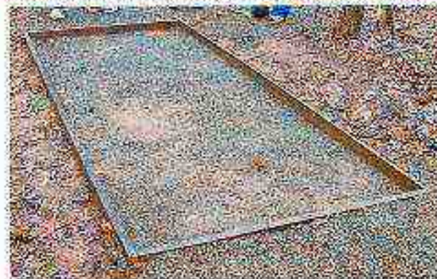
Frame is ready for concrete.
