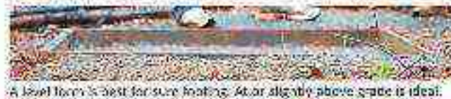
A level base is best for sure footing. 4" or slightly above grade is ideal.
