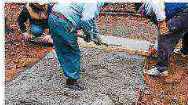
Once enough concrete is in the form, use 2x4 to screed, filling all areas.
