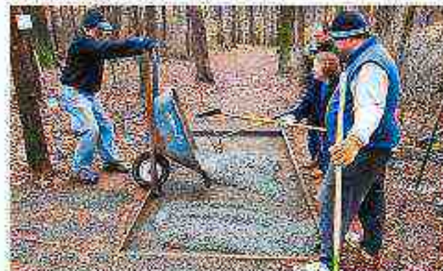
Use wheelbarrows to transport concrete to tees in remote areas.
