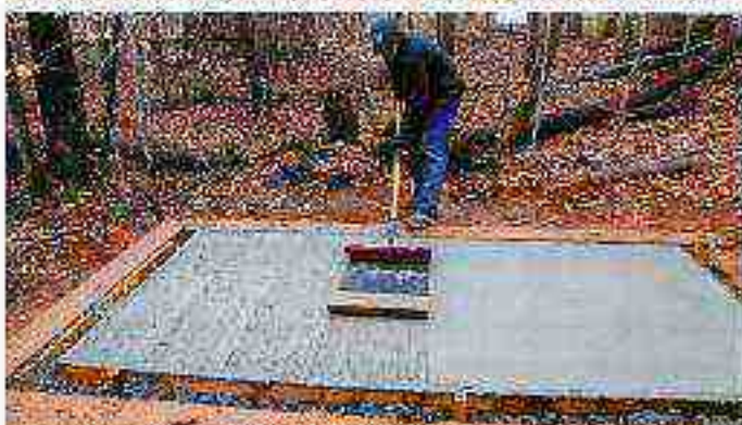
Drag the texturing tool across the pad from the side.
