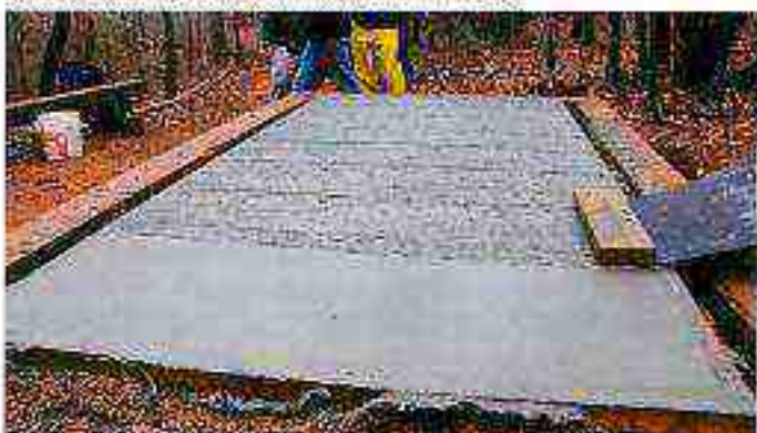
A close-up shows the difference between textured and untextured concrete.
