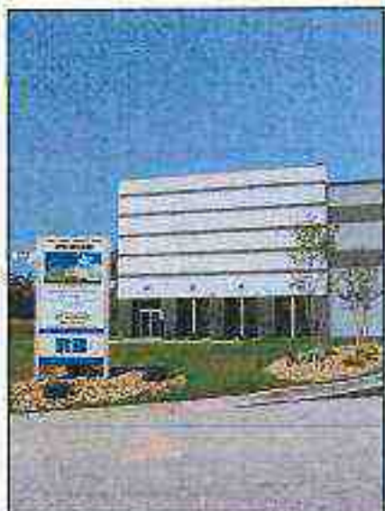
Available product, or lack thereof, was what Alexander advocated most. In 2011, Oconee County took ownership of a 50,000 SF Shell Building, located in the Oconee County Commerce Center. Referred to by one official as "the best Shell Building in South Carolina."
