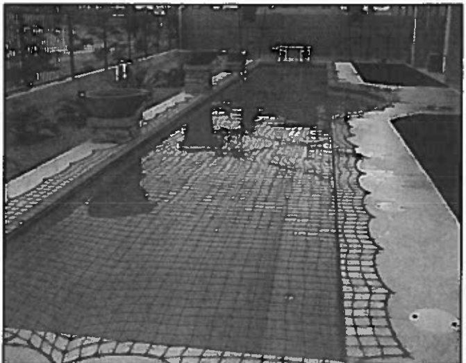
Commentary Figure 305.1(4) NONPOWERED MESH COVER DOES NOT ALLOW FOR ABSENCE OF BARRIER AROUND POOL
