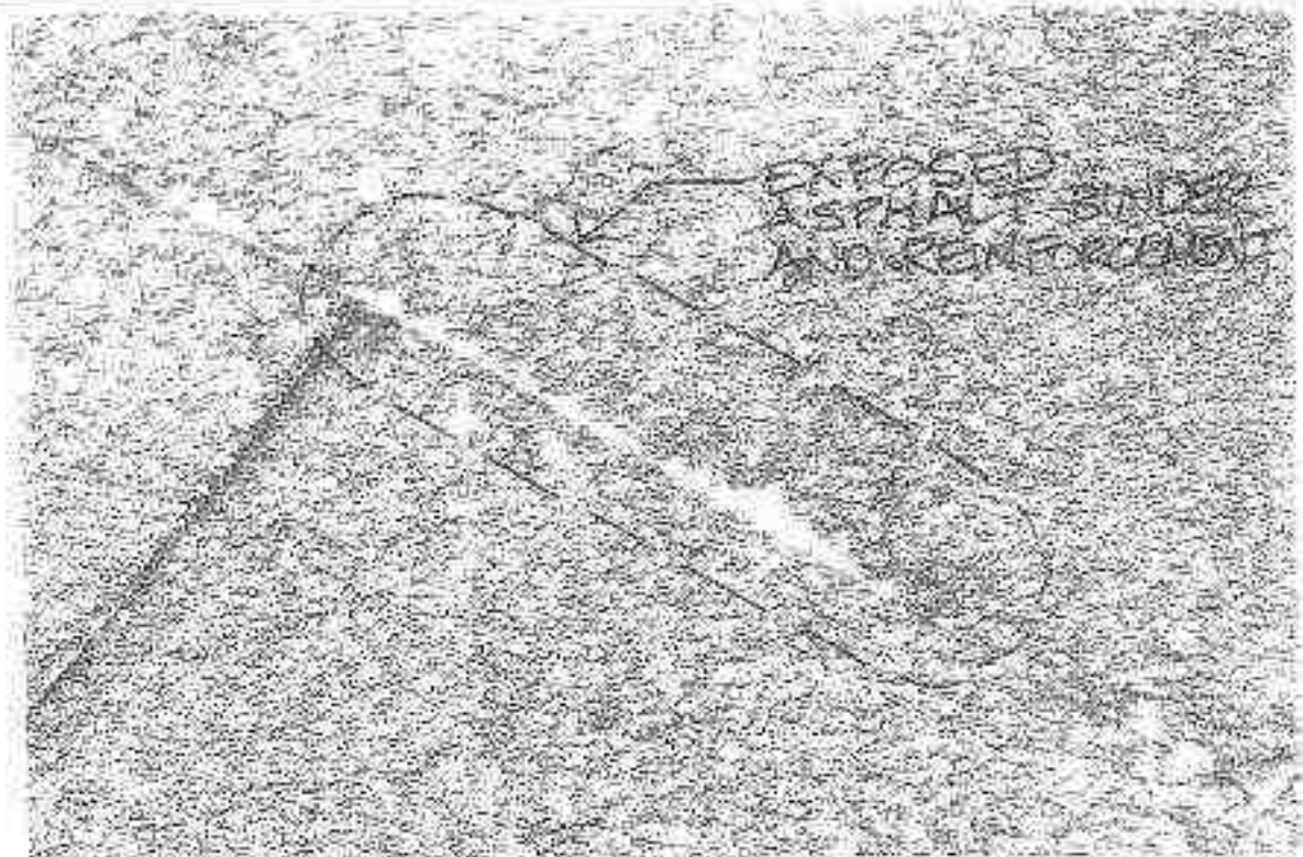
PHOTO 3A: View of exposed asphalt binder and fiberglass reinforcement on a typical shingle.
