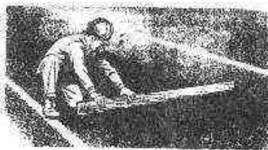
Figure VI—Straightedgeing the patch.
