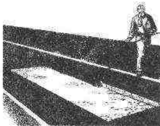
Figure 2—Applying tack coat to vertical surfaces
